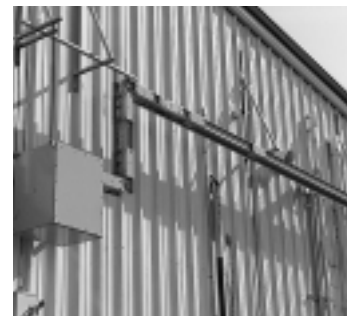
Complete outdoor run of Spectra Series Busway.
