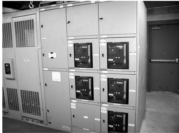
Figure 3. Low Voltage Switchgear Units
