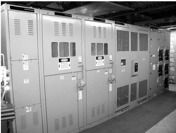
Figure 2. 500kVA Unit Substation
