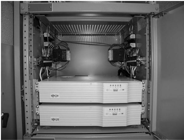
Figure 5. Redundant Uninterruptible Power Supplies
